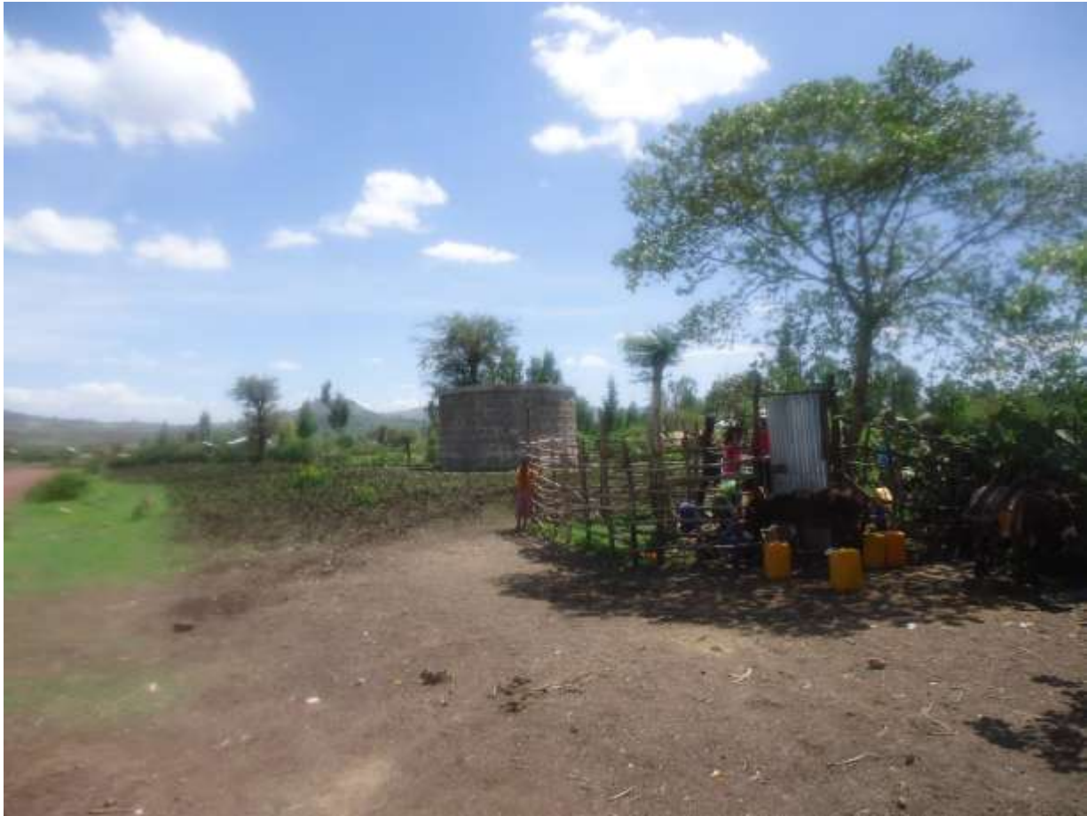
Figure 5-6: Potable Water Reservoir and distribution point in Abu Gerbi
