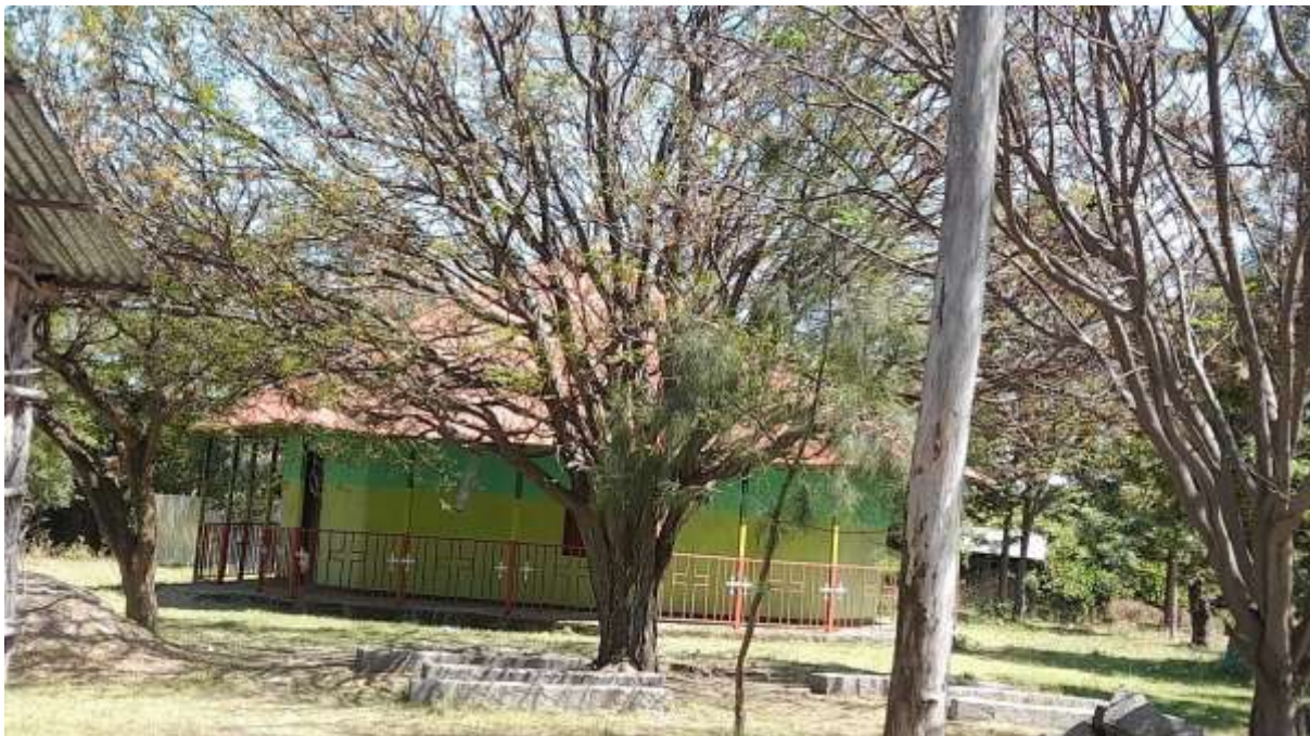
Figure 8-8: Orthodox Church within the project cite
